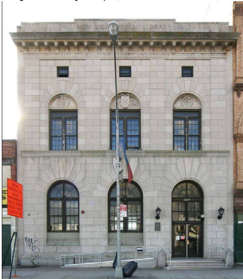
The New York Public Library, 125th Street, 224 East 125th Street, Main (North) Elevation. New York City Landmarks Preservation Commission The New York Public Library, 125th Street Branch Designation Report. Photo by Christopher Brazee, 2008.
