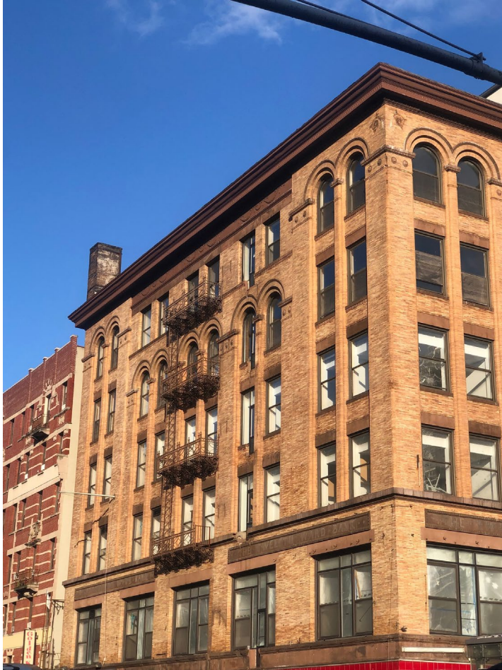
12th Ward Bank Building. Photo: Lorraine Colbert
