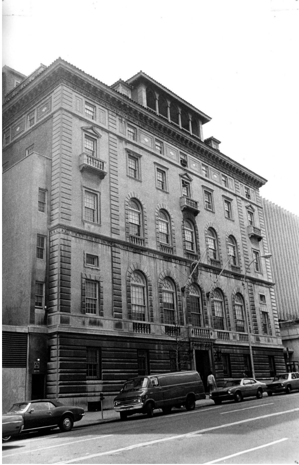
Casa Italiana, 1151 Amsterdam Avenue. Date: 1926-27. Architect: McKim, Mead & White. New York City Landmarks Preservation Commission Casa Italiana Designation Report.
