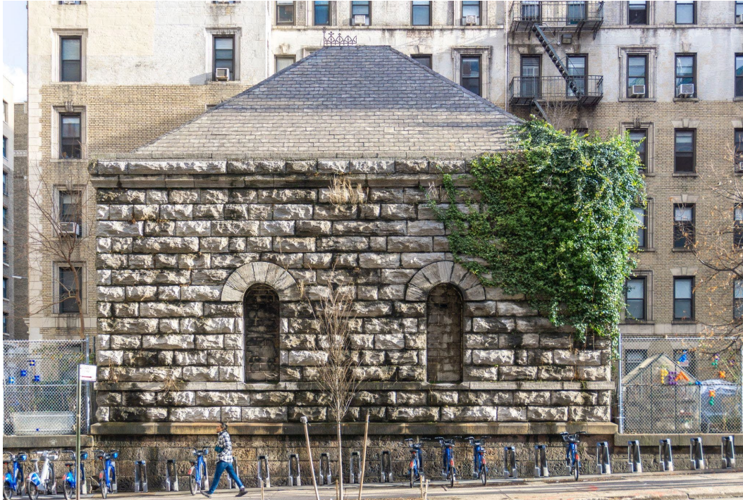
Croton Aqueduct West 119th Street Gatehouse. Photo by Lorraine Colbert
