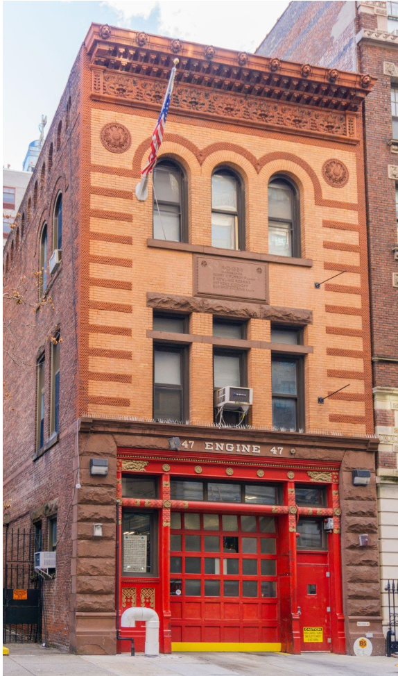
Fire Engine Company No.47. Photo by Lorraine Colbert
