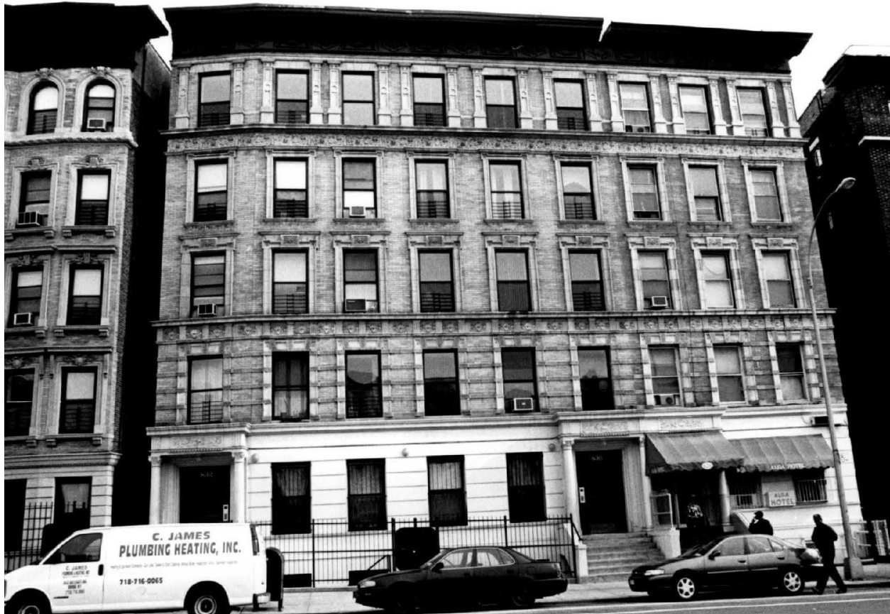
828, 830 and 832 St. Nicholas Avenue (aka 31, 33 and 35 St. Nicholas Place). New York City Landmarks Preservation Commission Hamilton Heights/Sugar Hill Northwest Historic District Designation Report. Photo by Carl Forster.
