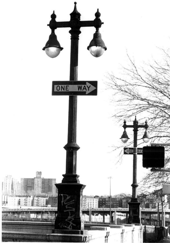
fig. 30. Special Iron Twin Standard. A special post, used only in this location at the entrance to the Harlem River Drive at Adam Clayton Powell Jr. Blvd. The original luminaires were octagonal lanterns. Landmarks Preservation Commission.
