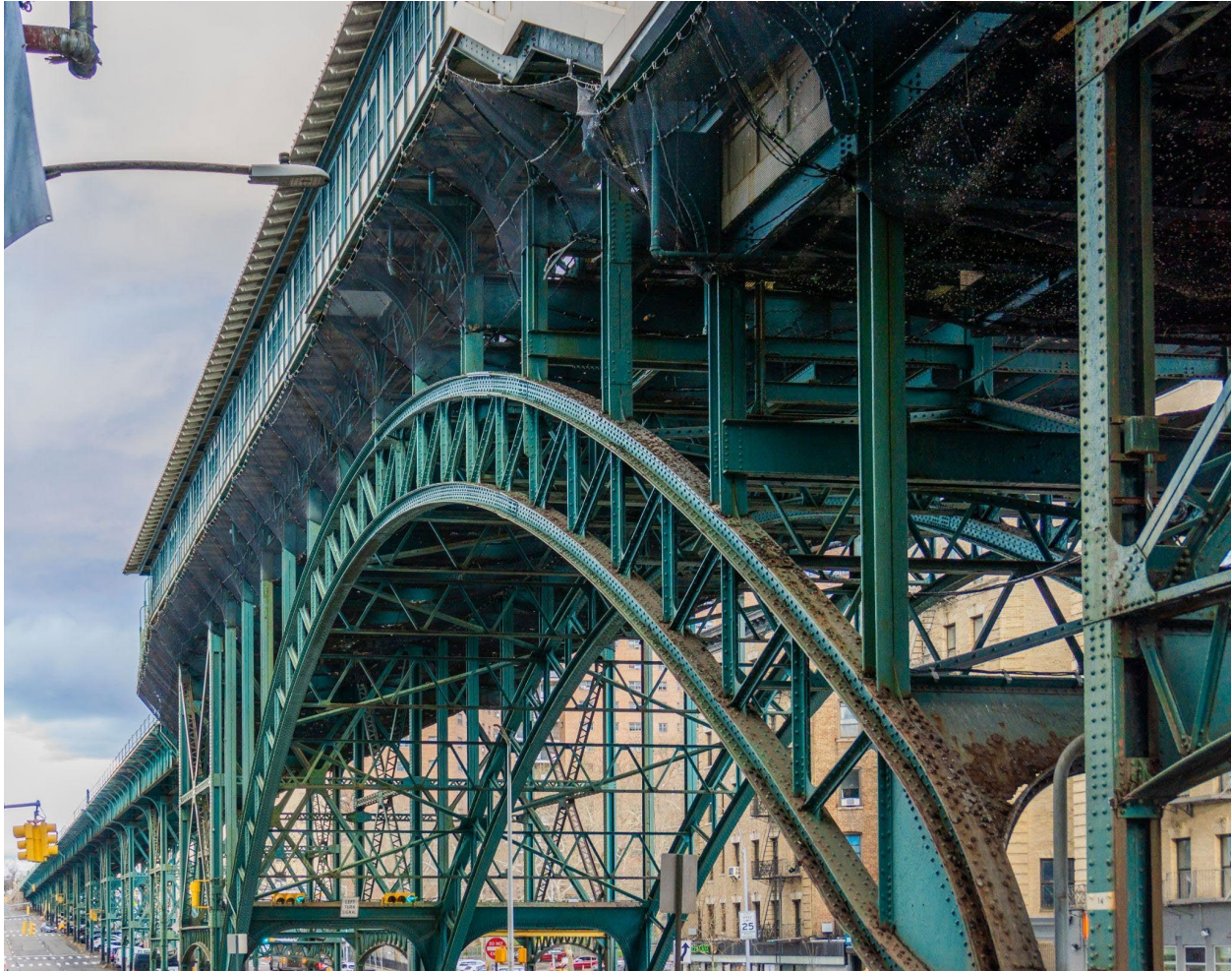
IRT Broadway Line Viaduct. Photo by Lorraine Colbert
