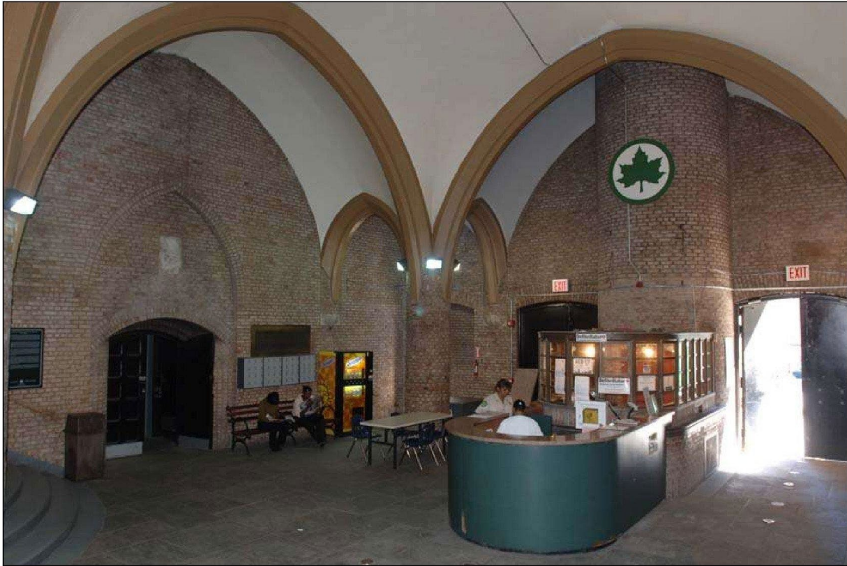
Jackie Robinson (Colonial Park) Play Center Bath House Interior: View Looking Northeast with Ticket Booth, Borough of Manhattan
