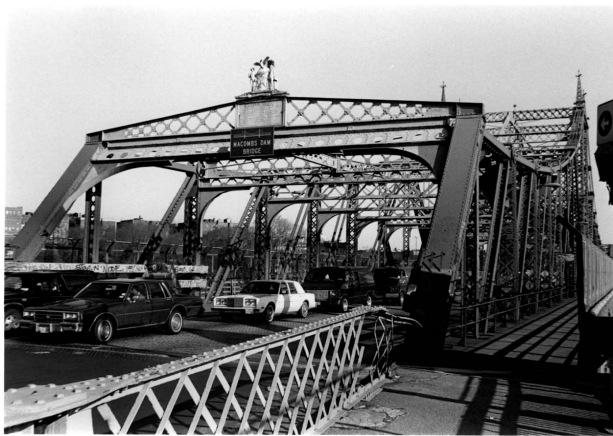
fig. M: Macomb's Dam Bridge, central swing span
