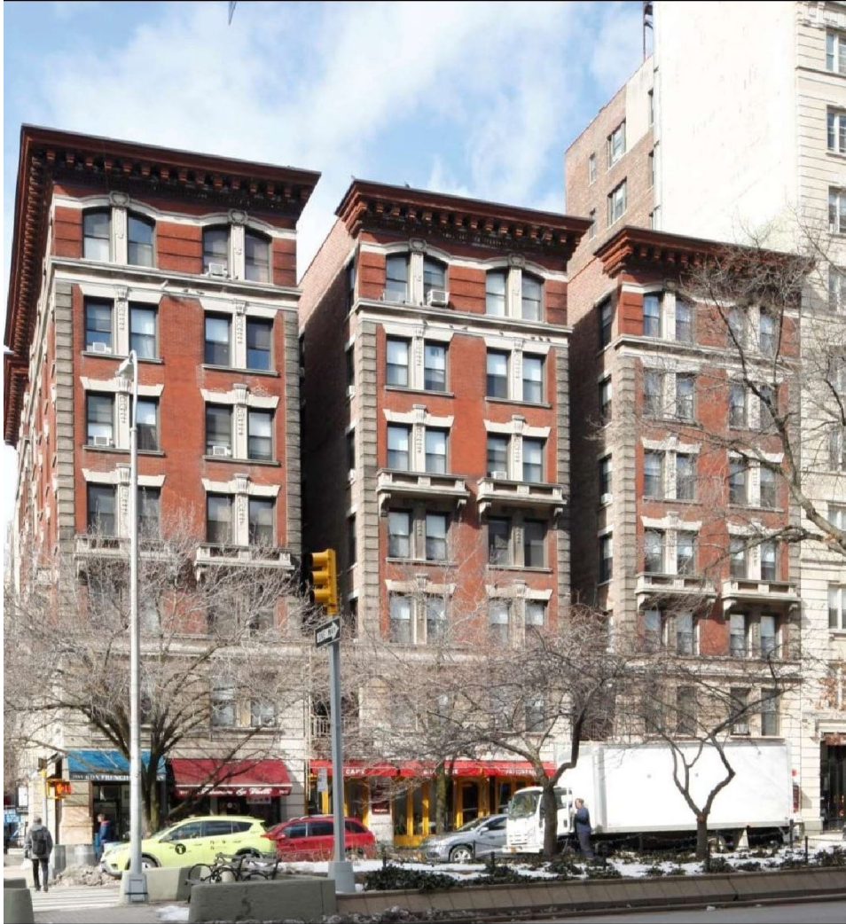
601 West 112th Street, George F. Pelham, 1901-02. New York City Landmarks Preservation Commission Morningside Heights Historic District Designation Report. Photo by Sarah Moses, 2017.
