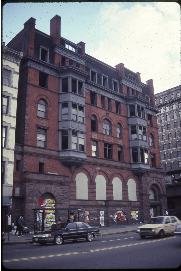
Mount Morris Bank Building February 1, 1991
