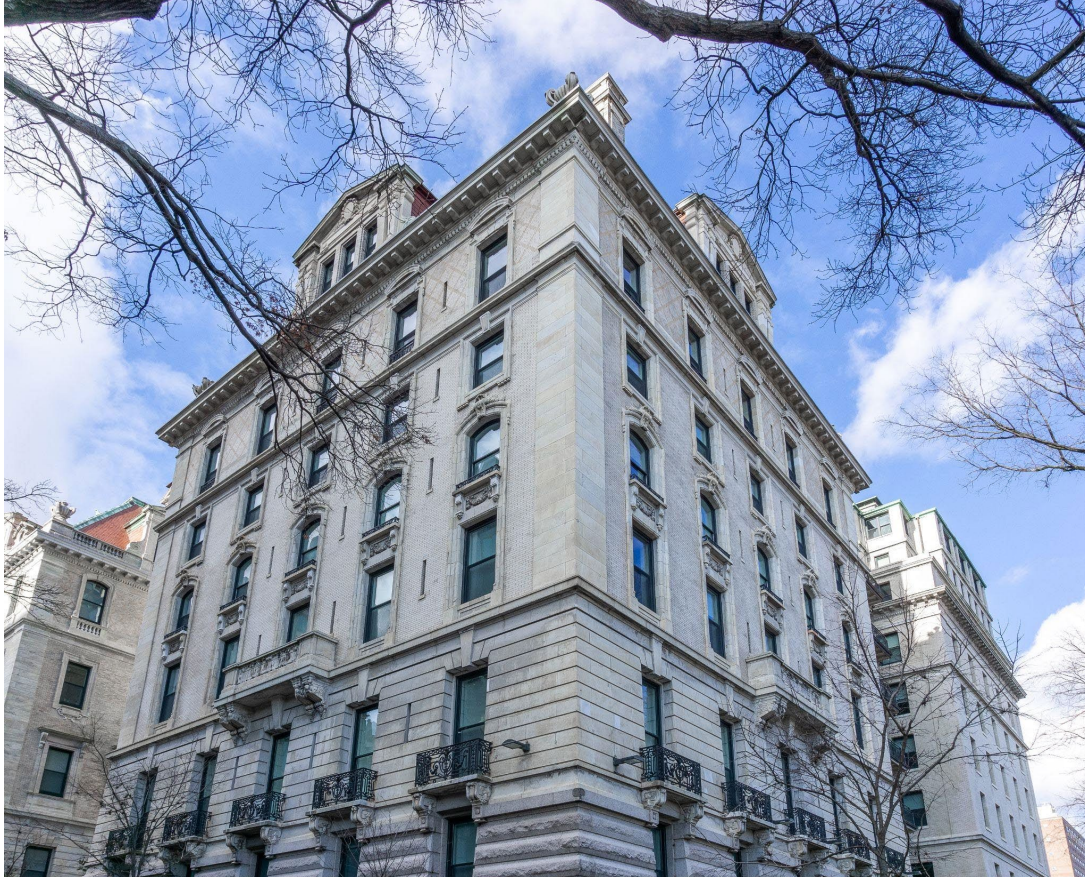
Plant and Scrymser Pavilions for Private Patients, St. Luke's Hospital. Photo by Lorraine Colbert
