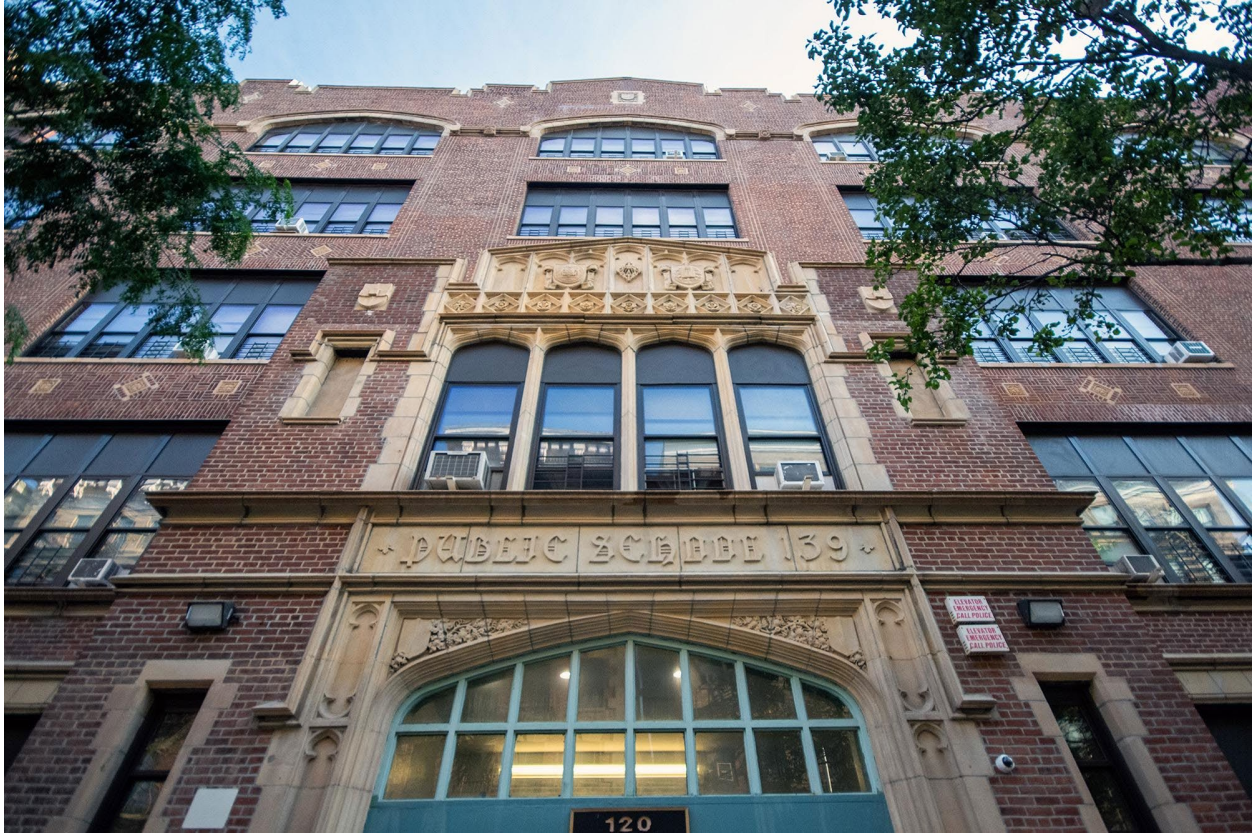
The Senior Citizen Apartment Building at former Public School 139. Photo: Melanie Nanez
